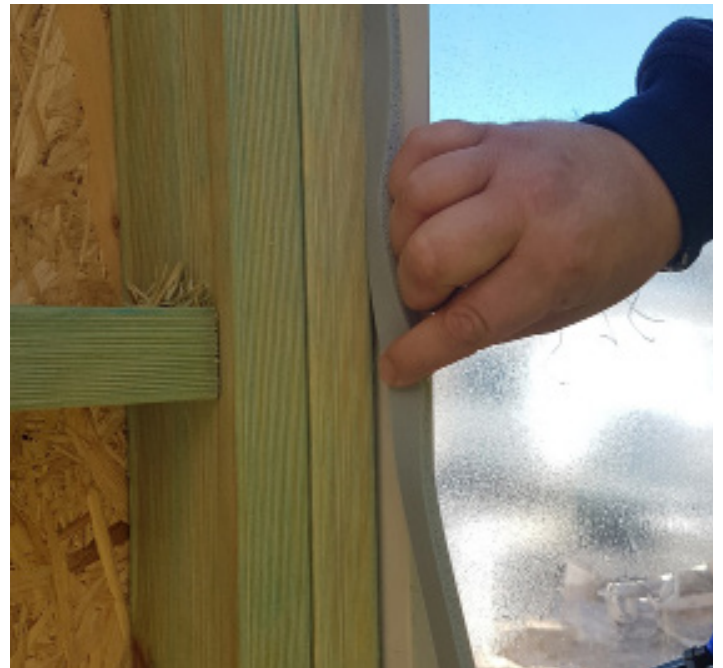
Figure 11 Applying high density acoustic foam
