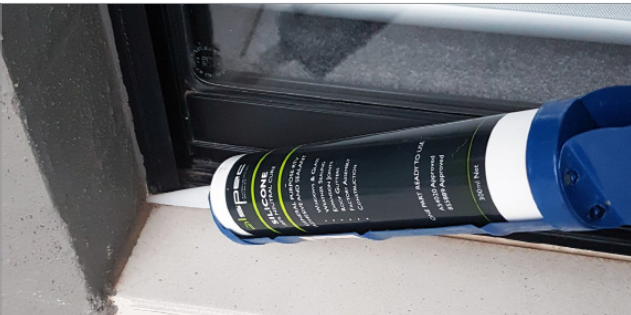
Figure 10 Applying sealant to the external frame of a glazed sliding door.
